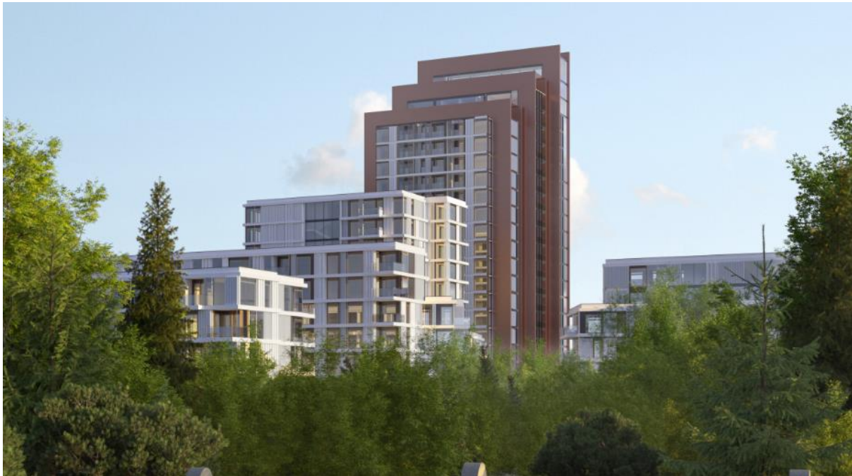
Figure 3: View of the development from the south, demonstrating the composition and height transitions proposed
