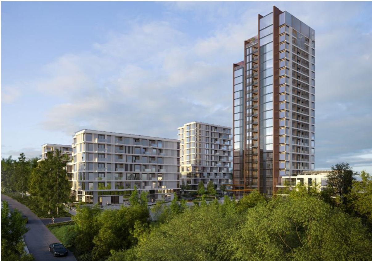
Figure 4: View of the scheme facing north along Golf Lane
