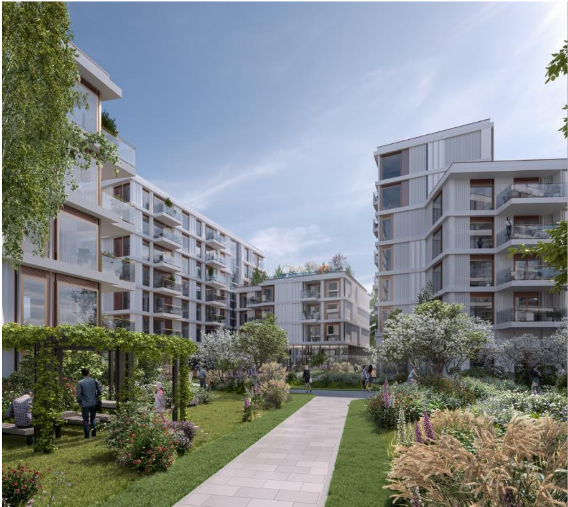
Figure 5: CGI internal view, demonstrating the environment that will be delivered within the centrally located communal open spaces
